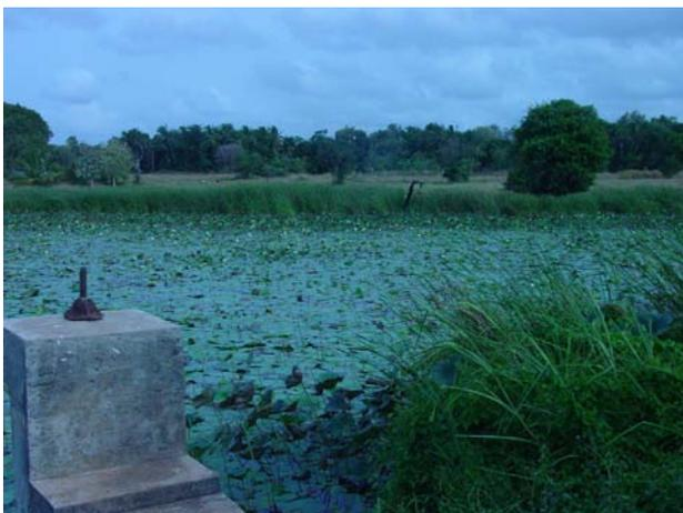
Picture 1: Small tank. Siltation is visible and is caused by soil erosion
